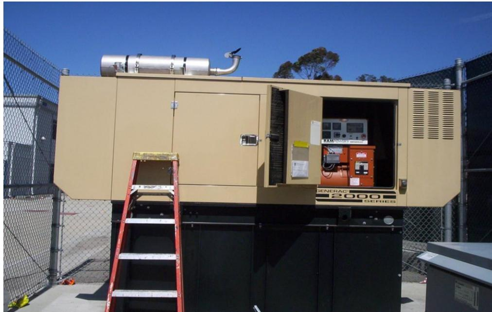
**Diesel Generator Retrofitted With A Particulate Filter**
